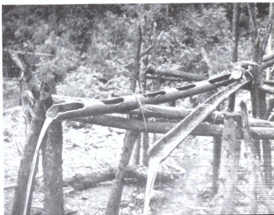
Water-line of bamboo pipes
